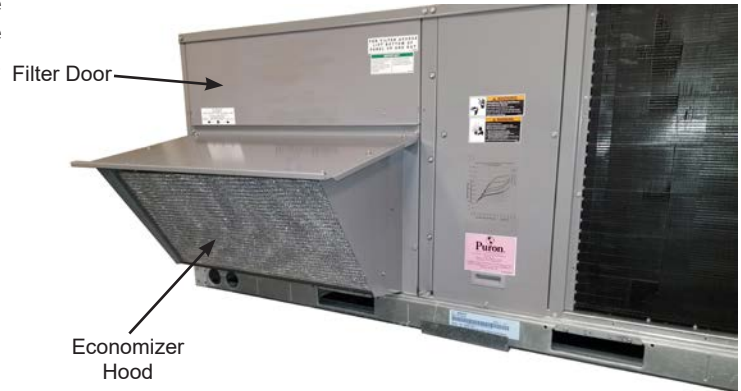
Figure 17 – Install Economizer Hood and Unit Filter Access Door
