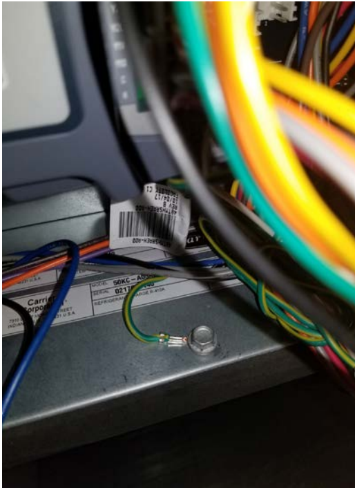
Figure 12 – Connect Ground Wire From Controller
