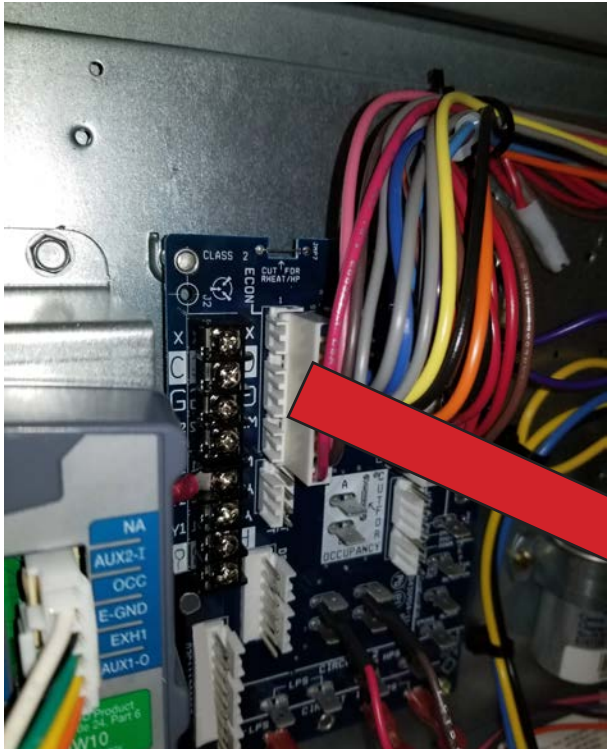
Figure 8 – Unplug ECON plug from Central Terminal Board (CTB)
