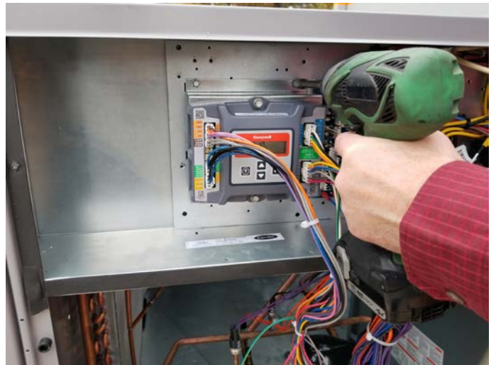
Figure 7 – Mount Controller Assembly in Unit Control Box
