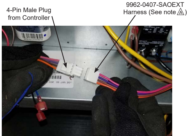
Figure 13 – Connect 9962-0407-SAOEXT Harness to Harness from Controller (See note )
